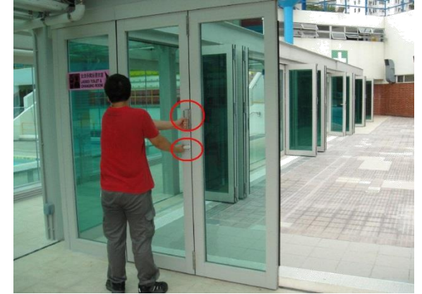
3) Pull door panels on left hand side toward to the middle for closing
