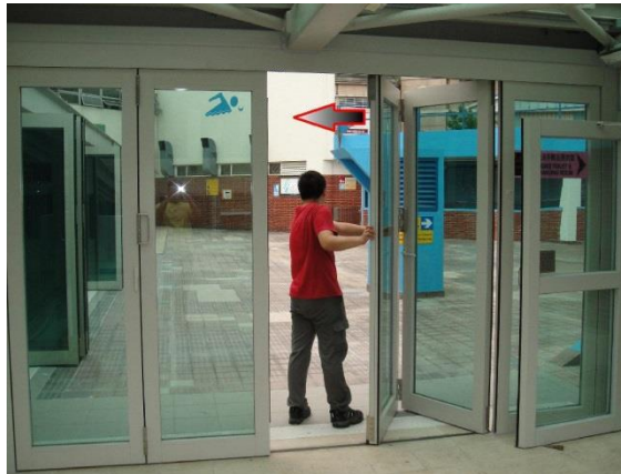
5) Pull door panels on right hand side toward middle.
