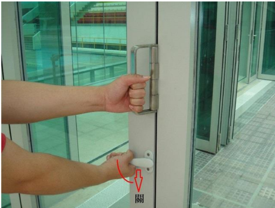
4) Turn the handle lock downward to lock the door.as above photo
