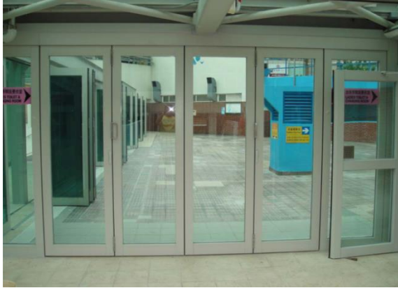
1) Bi fold Door in closing position
