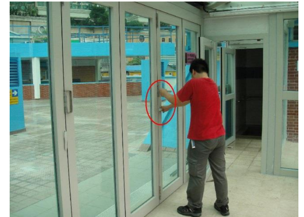
6) Pull the upper handle and use another hand to lock the door (as photo bellows)
