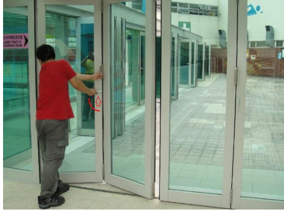
2) Turn the lower handle lock clockwise direction upward for opening showed as above photo
