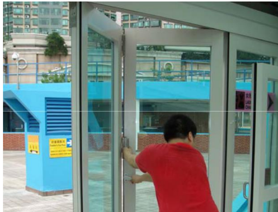
5) Turn the lower handle lock clockwise direction upward for opening
