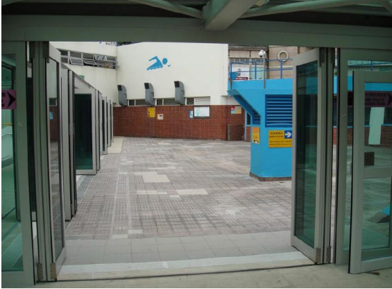
1) Bi fold Door in opening position
