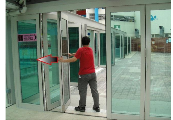
3) Push the door panels to the side as the above arrow shows to the left
